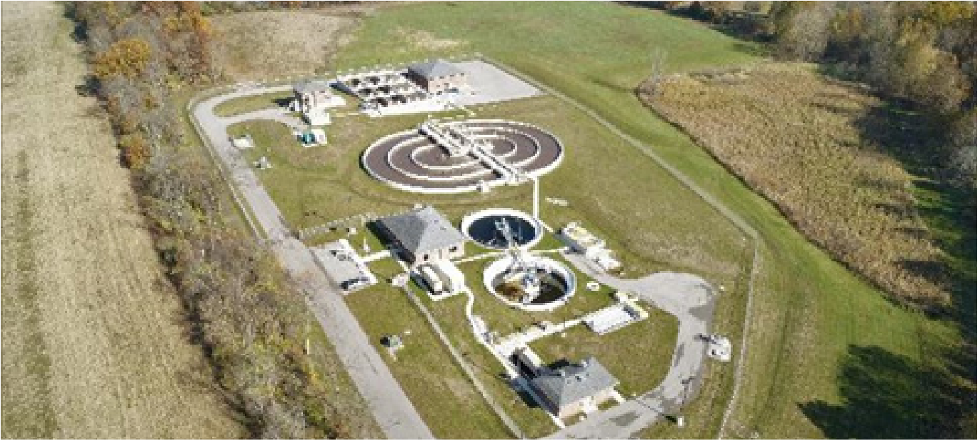
At the Huntertown, Indiana Wastewater Treatment Plant, Evoqua's Orbal® system was designed for 1.5 MGD with three reactors in series to support simultaneous nitrification-denitrification (SND) and meet an average phosphorus (P) removal limit of 0.44 mg/L.
